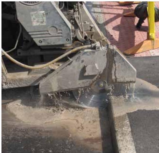
Cutting through the kerb stones and into ducts
