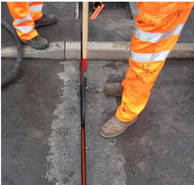
Installation of the 2 x 20mm sub-ducts
